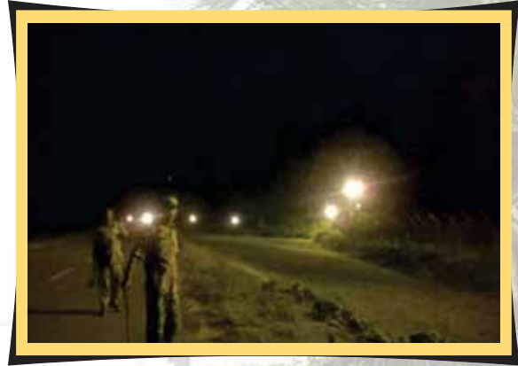
Flood Lighting Work in Tripura
