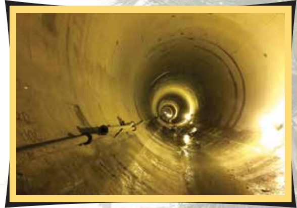
Concrete lining at HRT of New Hathiari HEP Unit-120 MW
