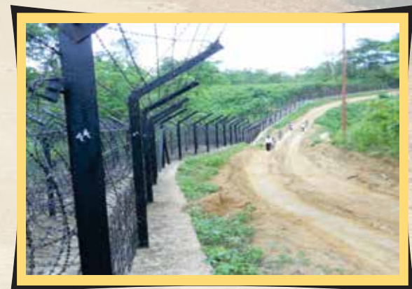
Construction of Fencing & Road Along IBB in Lawngtalai District of Mizoram
