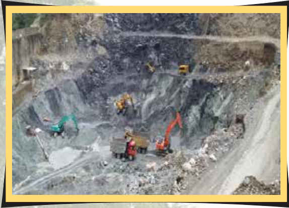
Excavation at Power House Area at 120 MW, New Hathiari, HEP Works
