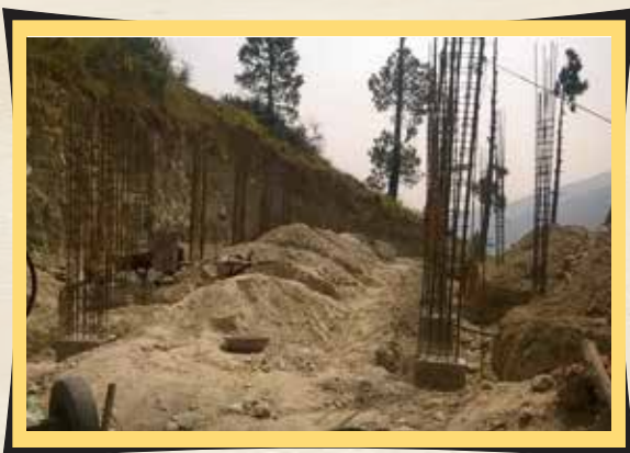
Casting of Column at Rusa Works, Bhikiyasain
