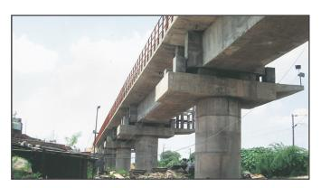
involving launching of Pre-stressed box girder of 25 meters span each weighing 250 MT and also constructed elevated Railway Station. NPCC in past successfully
