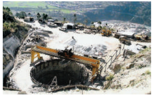
Surge Shaft at Maneribhali Hydro Electric Project, Uttarakhand
