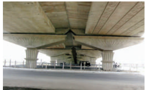
Flyover at Greater Noida Expressway, Noida
