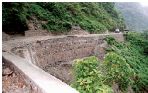
Hathiari Road Works, Protection Wall
