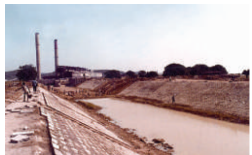
Power Channel in Anpara Thermal Power Plant, U.P.
