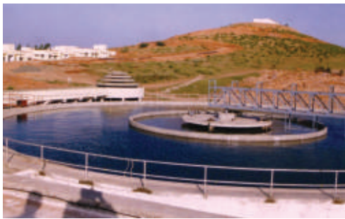
Water supply works at Bagalkot, Karnataka
