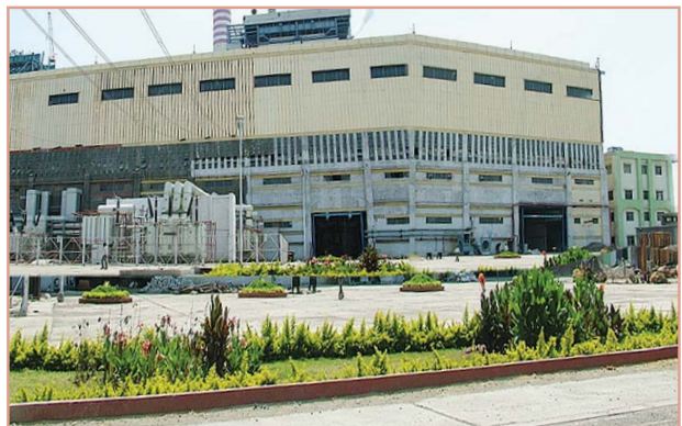
New Parli Thermal Power Station
