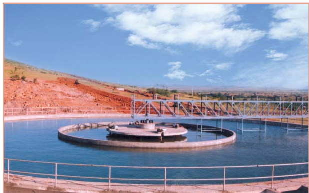
Water Treatment Plant, Bagalkot, Karnataka
