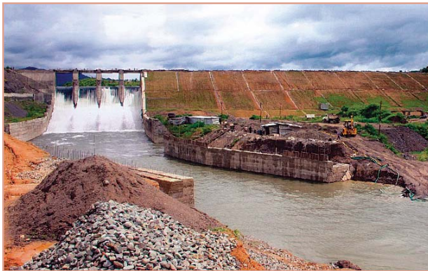
Khunga Dam, Manipur
